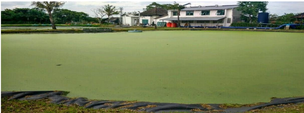
Figure 2. Existing Condition of Pond Outlet WWTP ITDC Nusa Dua Bali Algae Contaminated
