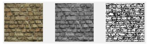
Figure 2- a view of bricks with not much of the similar textures, the left image has marked by the classified texture and the black pixels are those which have not been put under any clusters. those are typically related to the edges or higher frequencies.
